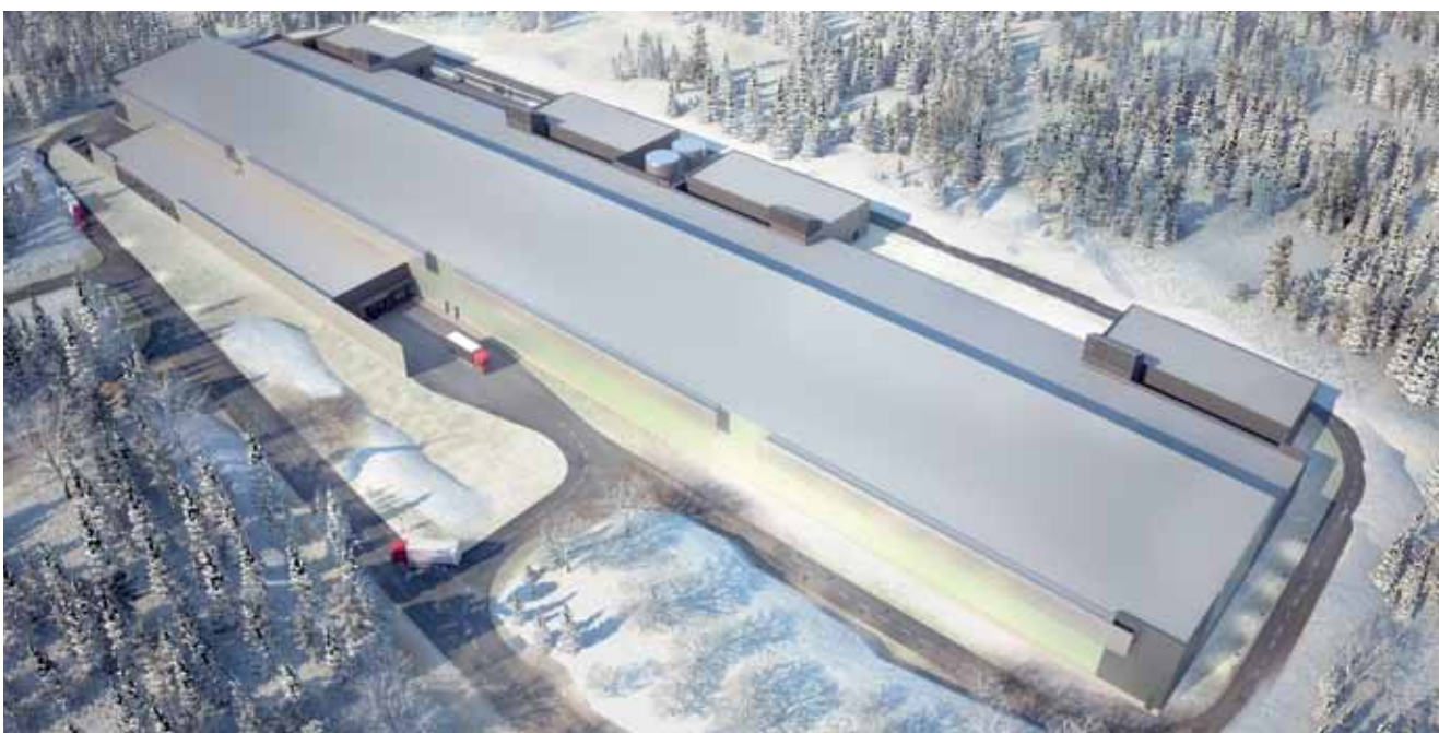
Facebook's new data centre in Sweden.
